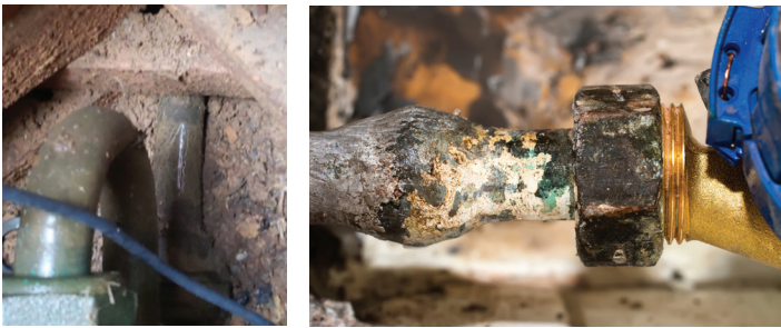
Lead pipes are wider at the base and can form a bulb.
