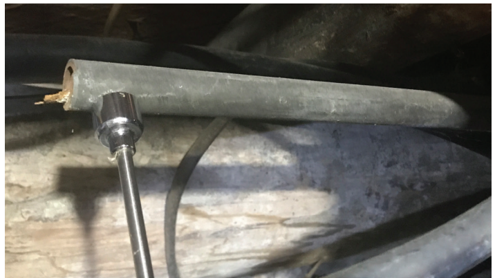
Lead pipes are wider at the base and can form a bulb.
